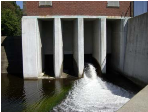
Lake Hopatcong sluice gates
