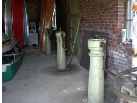
Hand cranks control sluice gates and fountain
